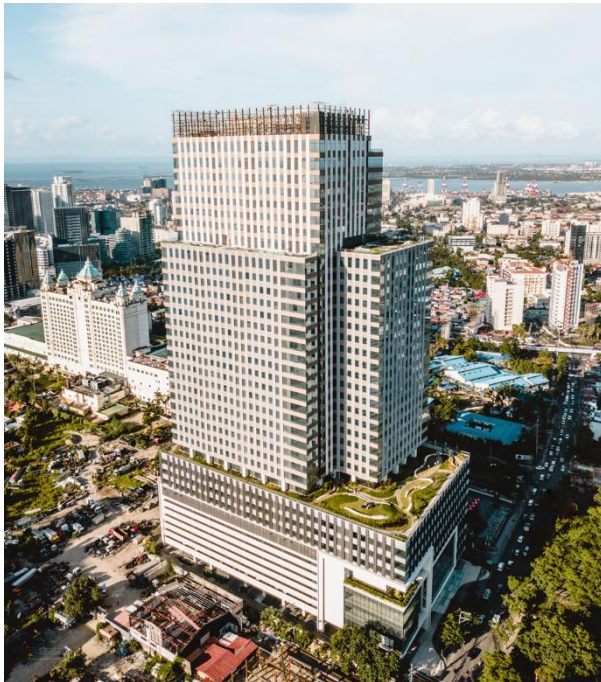
Cebu Exchange Exterior Façade
