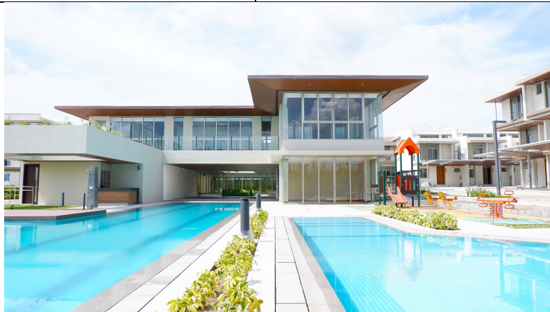
Sevina Park Villas, Villa Type B Model Unit and Neighborhood Pavilion
